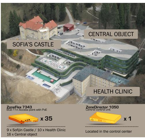
With implementation of 35 ZoneFlex 7343 Access Points and a central control unit Zone Director 1050, we were able to provide a powerfull and highly reliable Wi-Fi signal throughout the whole  $20.000^\circ$ m of the complex.
